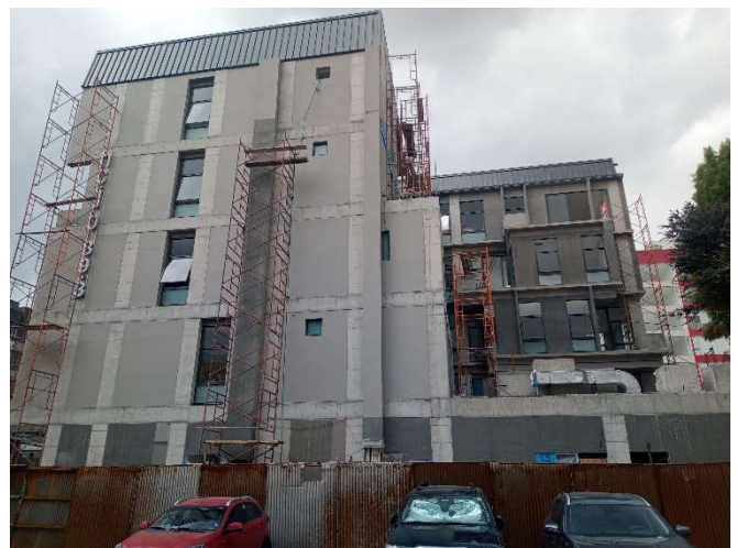
The new studio building is nearing completion.
