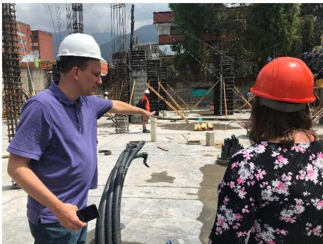
Geoff and Tammy at the building site
