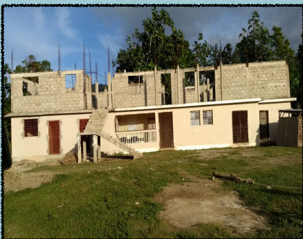
Construction progress update on the seminary. First floor exterior almost complete.
