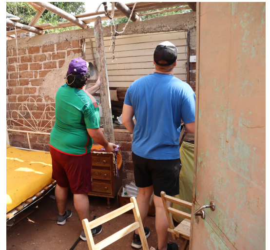
Replacing the roof on a very modest home of Cru staff
