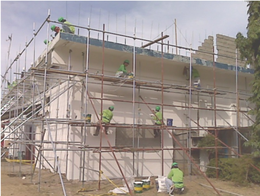
Renovations Under Way at Iba Transmitter Site
