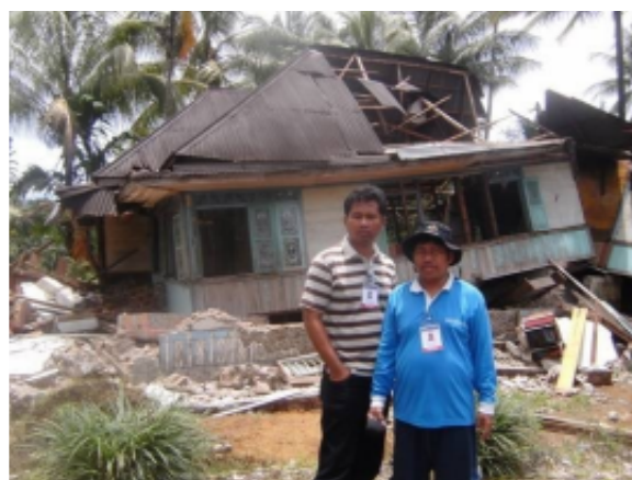
Earthquake Damaged Home
