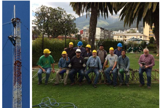
Tower removal crew
